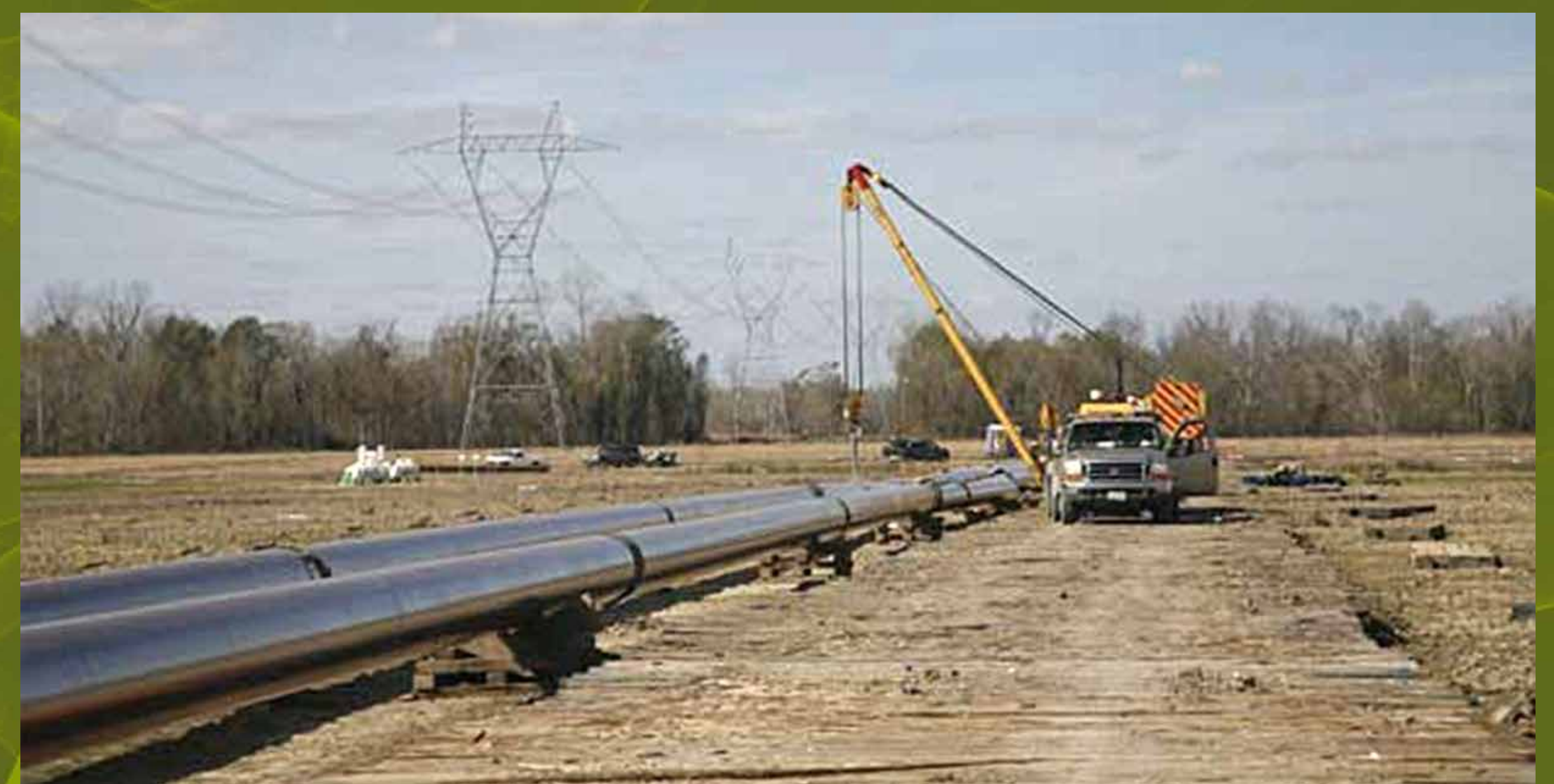
CO 2 pipeline. Denbury's Green Pipeline was designed to transport both natural and anthropogenic CO 2 and is routed near several potential industrial CO 2 sources. 2
